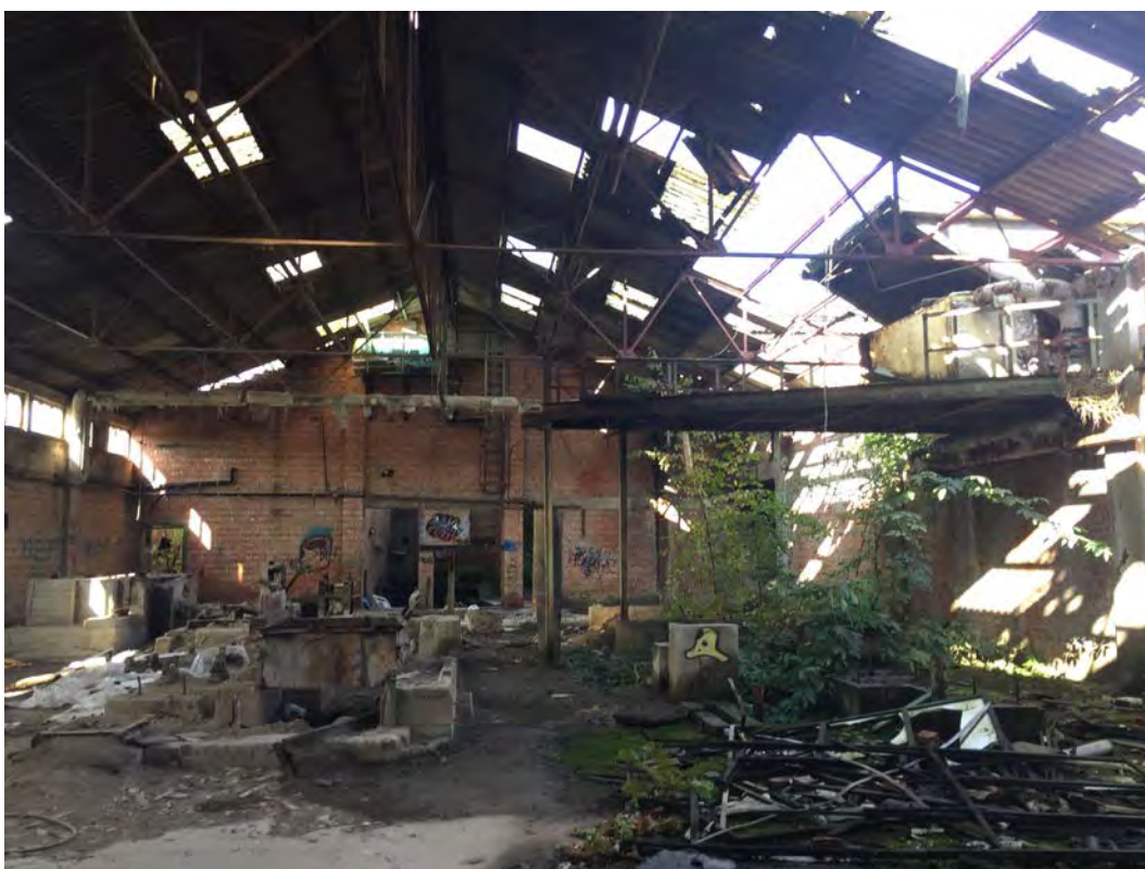
One of the abandoned production halls on site
