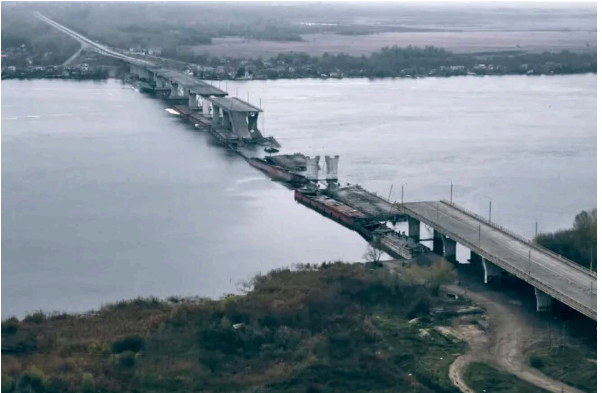
The destroyed Antonivsky Road Bridge over the Dnieper River in Kherson, Ukraine. Photo credit: © LIBKOS/AP].
