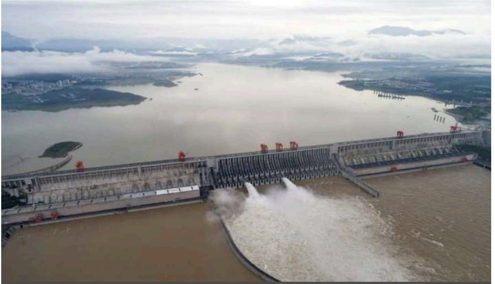
Three Gorge Dam China. Image credit © AP
