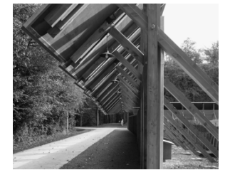
fig. 15. leper, Belgium, constructed in 2020 by Schenk Hattori.
