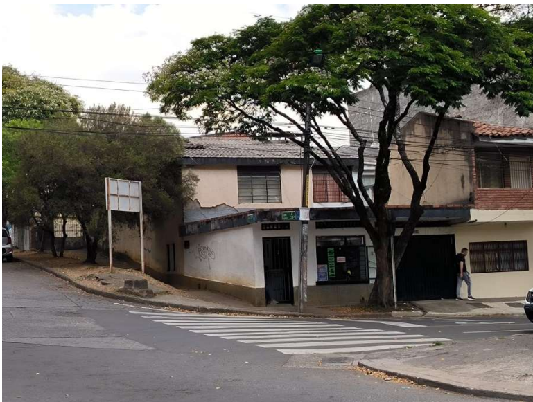
Fig. 3: Existing buildings on site. Picture: Cesar Salmona
