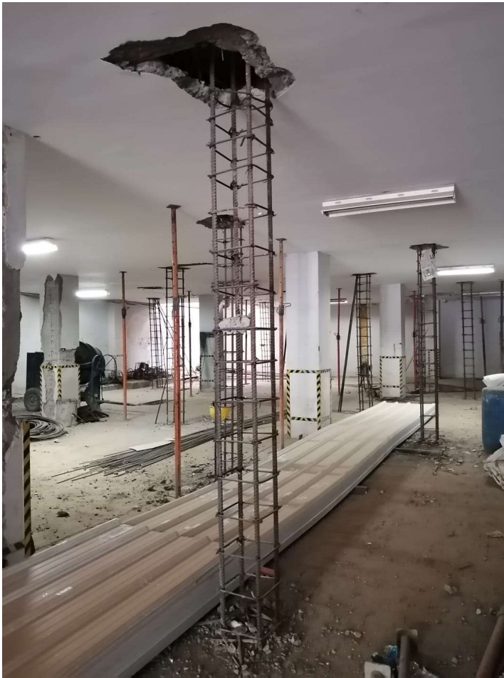
Fig. 5: Example of available technologies to react upon: references sent by the local building contractor. Picture: Cesar Salmona.
