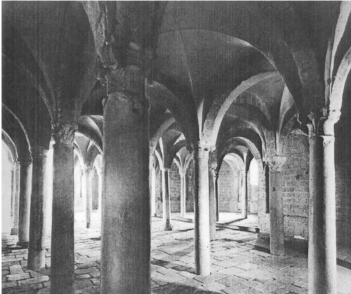
The crypt of San Pietro, facing northeast, with view of apse. (Parlata and Romano, Italia Romanica)
