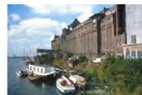
WEST FACADE FROM THE HOUTHAVENS' SOUTH-EAST CORNER (pic 9-95 /to N) Only from the Houthavens can the huge length of the old Silo be appreciated
